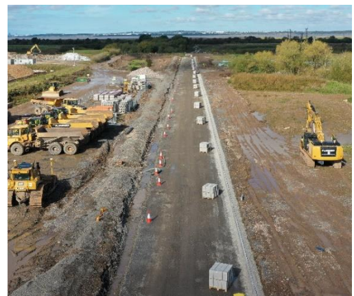
Image 02: Showing Road 1 Construction
