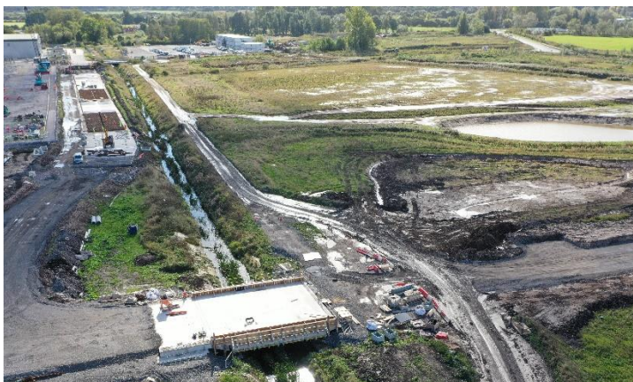
Image 01: Showing Road 4 Progress and West Central Drain Bridge
